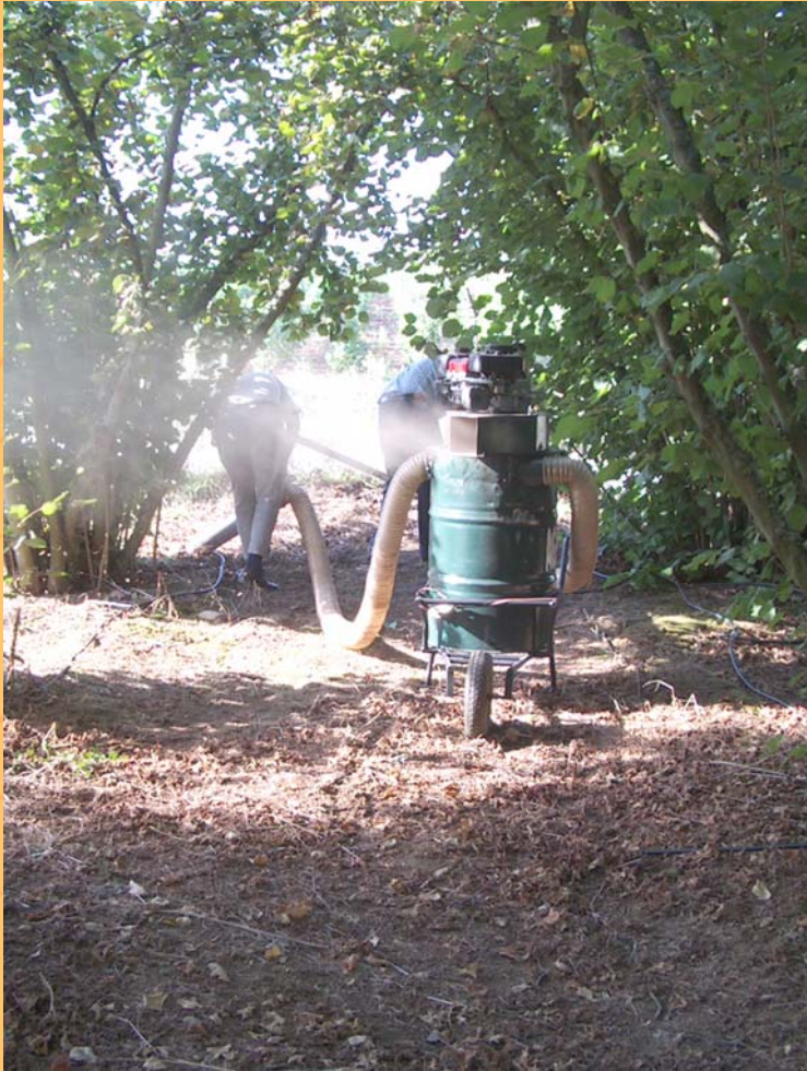
Material not stripped
